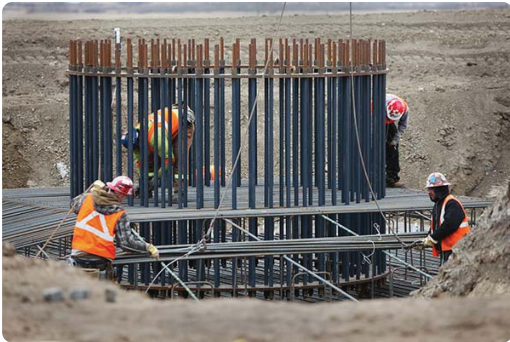
Constructing a wind turbine site for Halkirk Wind in Alberta.
