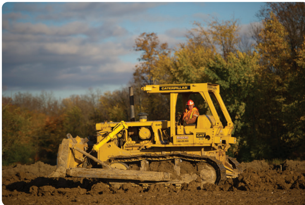
Beginning construction of Port Dover & Nanticoke, ON
