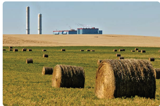
Genesee Generating Station, AB
