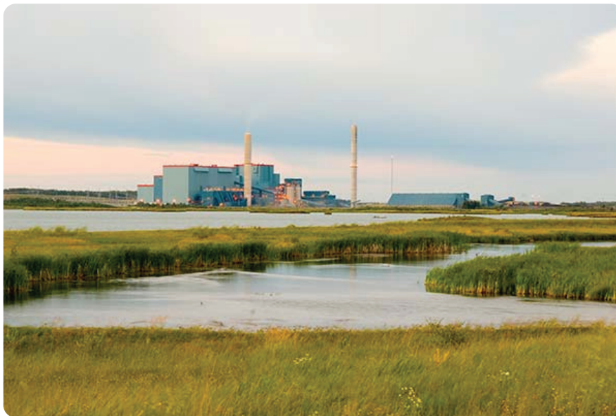
Genesee Generating Station, Warburg, Alberta
